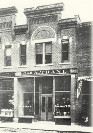
Trane Storefront La Crosse, Wisconsin 1891
